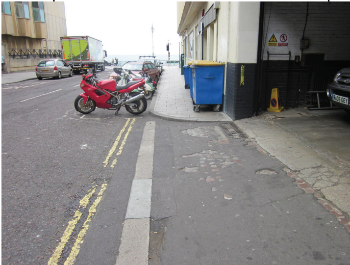
12. Ship Street. The southern end of the Old Ship car park needs a dropped kerb.
