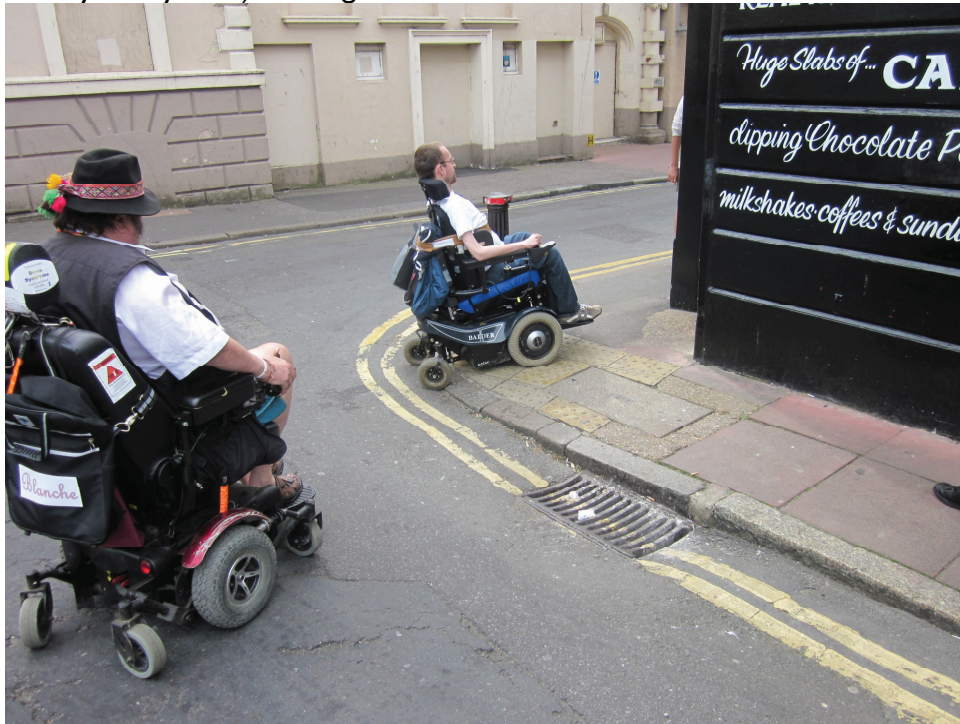
9. Middle Street. Dropped kerb at middle St / Boyces street junction (outside choccywoccydoda) is not good, hard for wheelchairs to use it.
