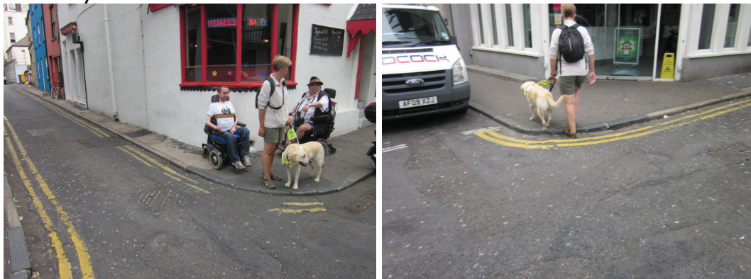
10. Middle Street. Dropped kerb required at Middle Street / South St junction. Currently forces wheelchairs on to road.
